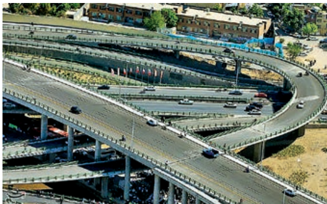
Urban Infrastructure - Imam Ali Highway
