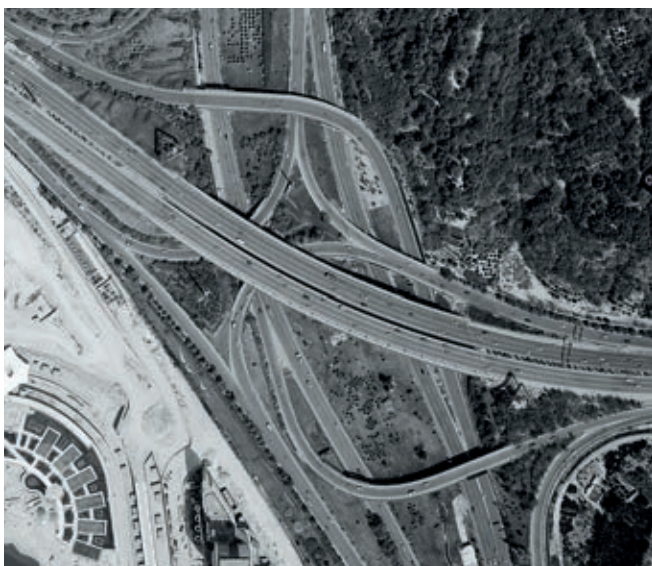
Fajr Bridge - Tehran
