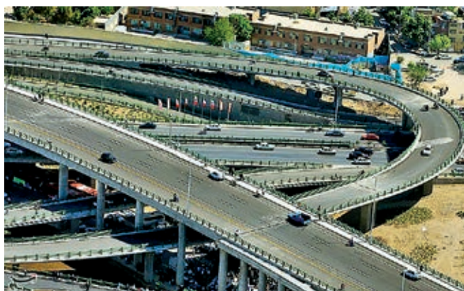
Urban Infrastructure - Imam Ali Highway
